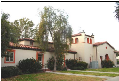
Language Arts Building Renovation at LAC
