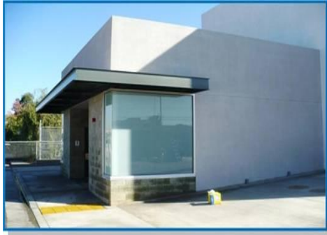
Central Plant at PCC
