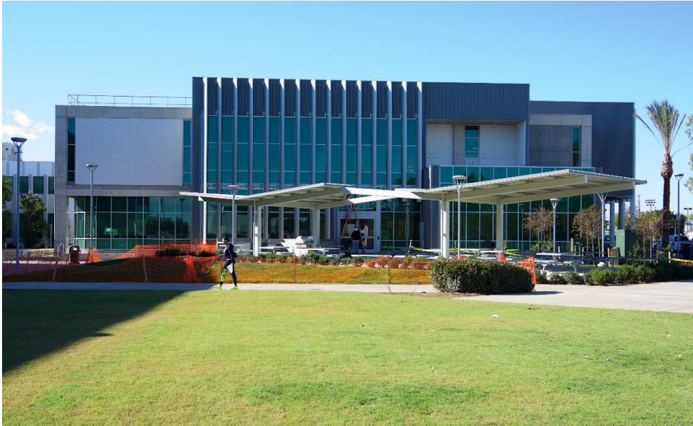
NEW STUDENT SERVICES CENTER – BUILDING GG AT PCC
